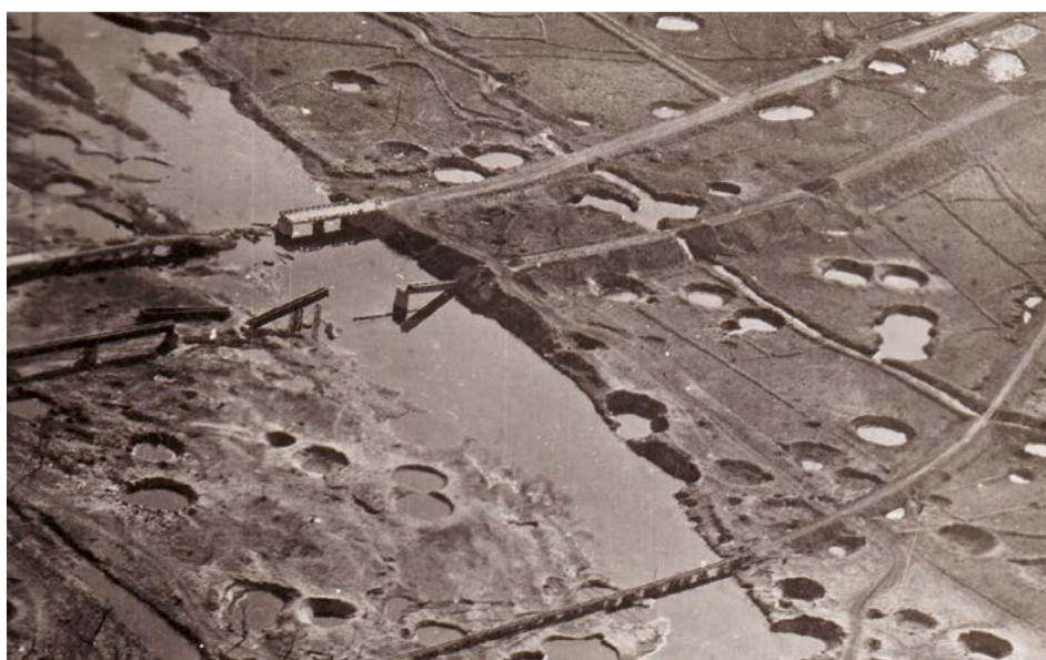
"Bomb damage around 3 bridges. Targets we knock down as fast as they re-build them".
