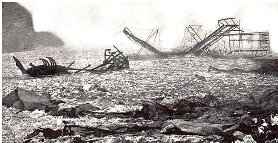
The burned out wreck of SSZ10 at Willingdon Hill Farm.
