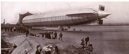
HMA No1 leaving its floating shed at Cavendish Dock, Barrow-in-Furness.
