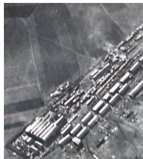
The repair sheds at Rayak, 28 February 1917, taken from 7000 feet.
